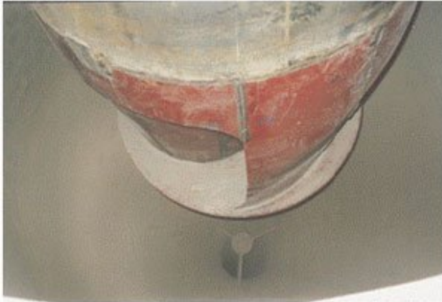
Installed HURRIVANE® at Mokrá plant
