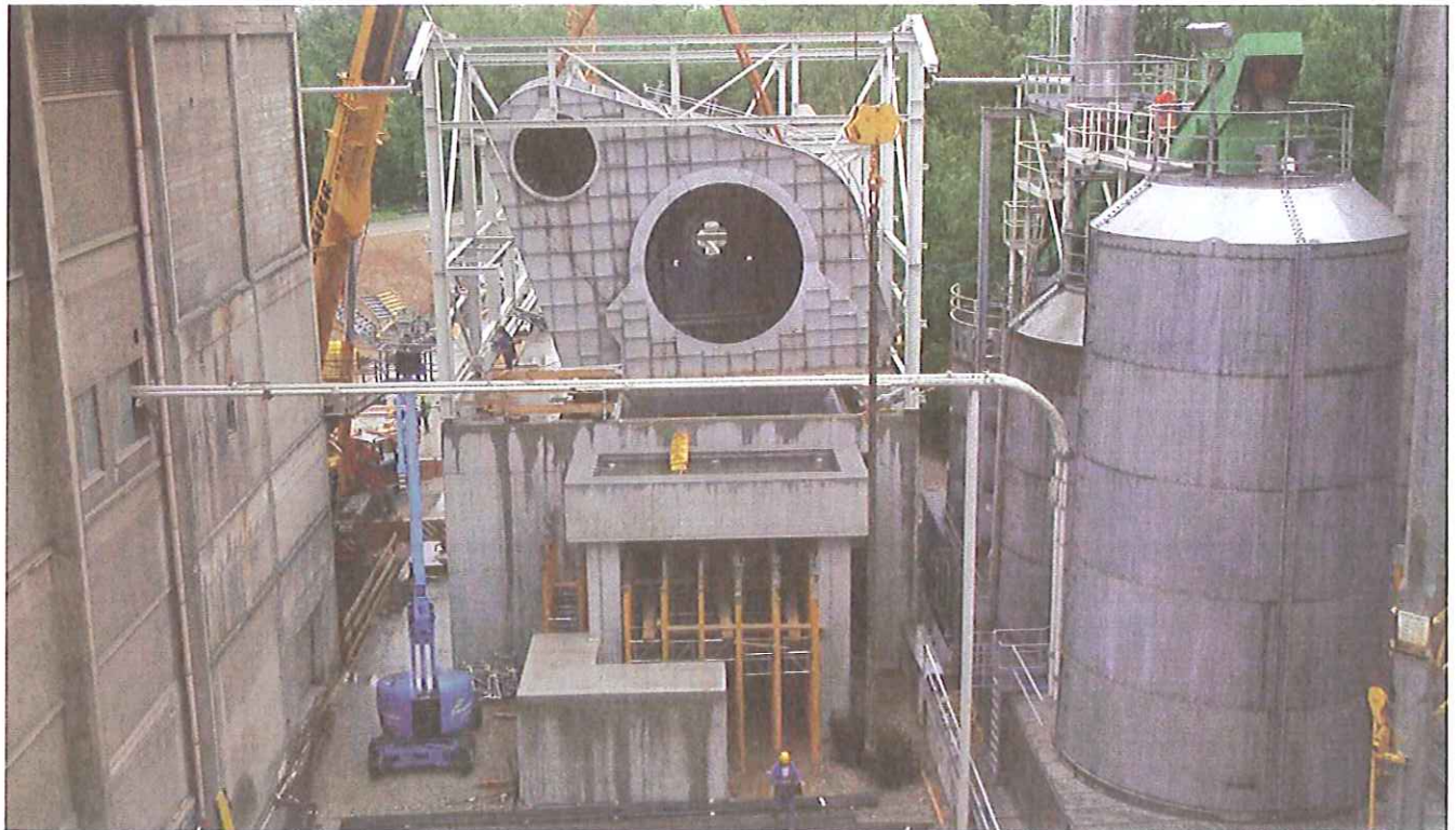
2 Installation of the kiln hood • Installation des Ofenkopfes
